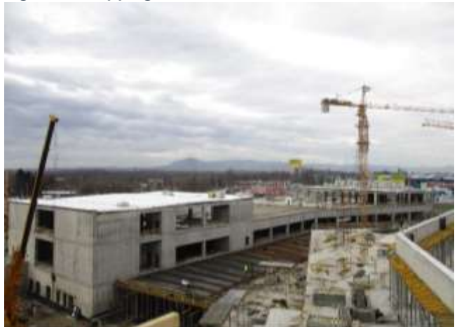
Figure 6: Shopping center Z construction site
